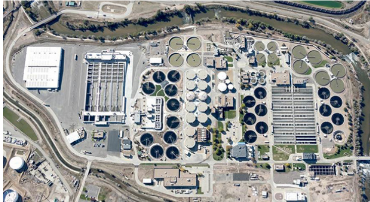
Figure 2. The Robert W. Hite Treatment Facility
