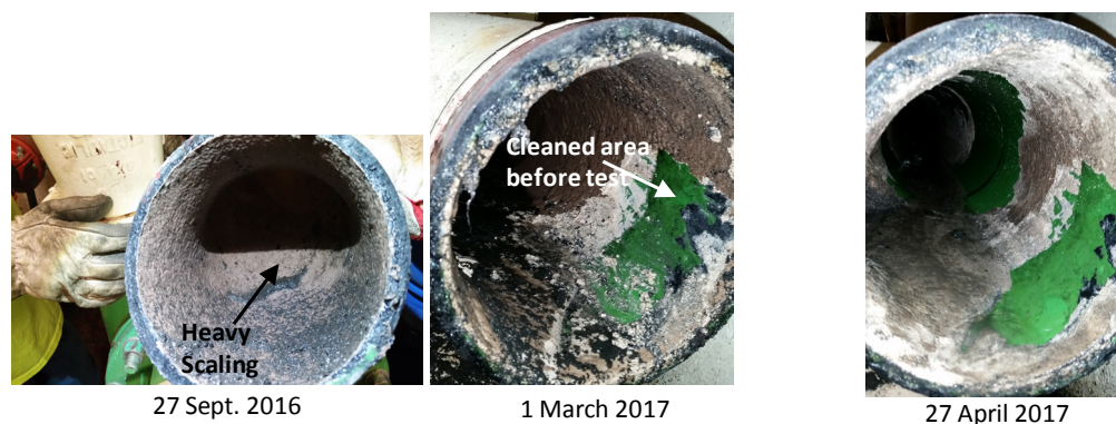
Figure 8. Before and After Photographs of the Transfer Pump Discharge Pipe
