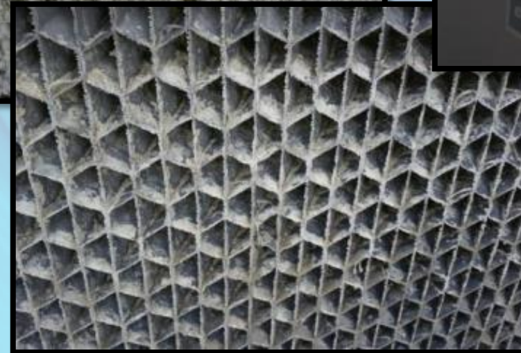
Drift eliminator after.
