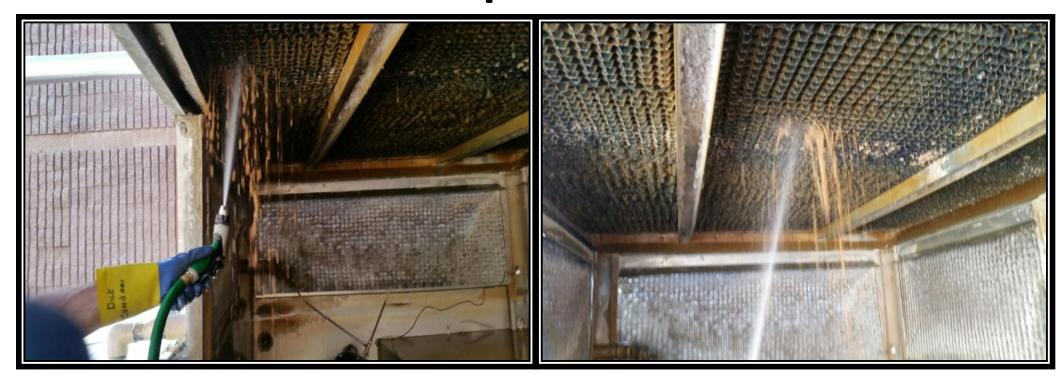
Instead of the hard scale that typically accumulates inside the cooling tower, loose brown mud-like material was found. A garden hose was used to easily remove the mud-like substance from the fill material and the drift eliminators.
