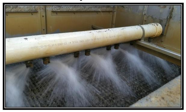
Due to equipment malfunction, the cooling tower's conductivity meter read 14,000  $\mu$ S, which was 6 times too high. Airman Payne repaired the damaged system and reset the controller back to the normal operational parameters of 2,300  $\mu$ S. No significant hard scale or bio buildup was observed on the nozzles or infrastructure.
